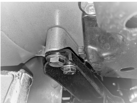
Installed forward support bracket:
